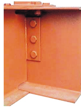
Fig. 2. Bolted shear connection – realisation
