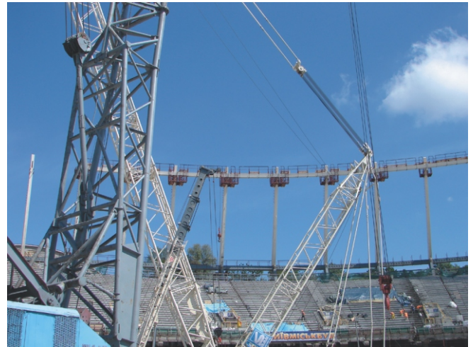
Stadium under construction
