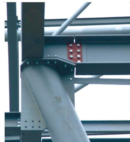
Fig. 5. Detail of the column end; connection between the column and girders
