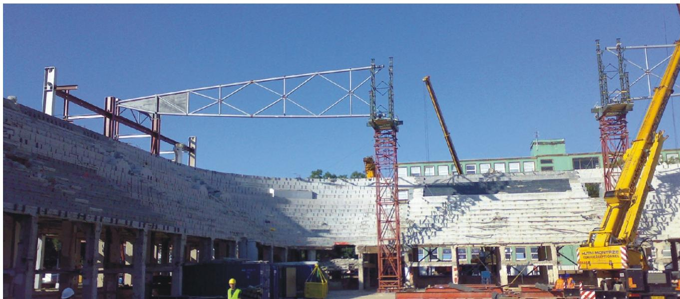
**Fig. 11:** Erection of the truss girder on the preliminary supports
