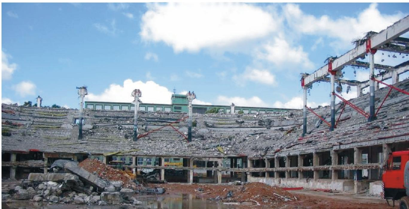
Fig. 3. Dismantling of the RC slab and columns
