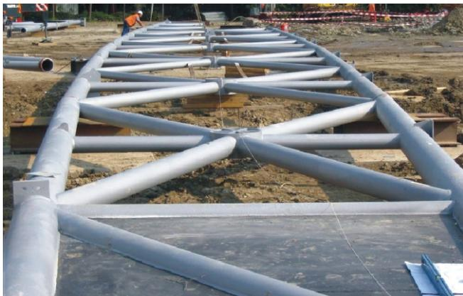
Fig. 8. Truss girder with total length of 86.0 m
