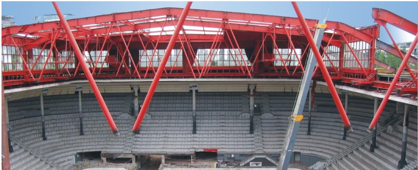
Fig. 2. Dismantling of the steel roof structure
