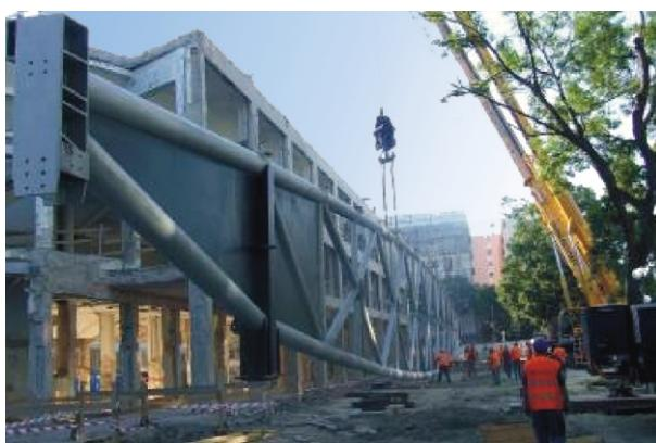
**Fig. 12.** Erection of whole truss girder by cranes
