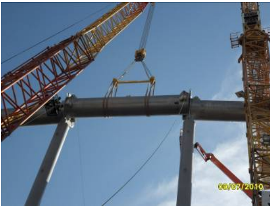
Fig. 9. The closing ring
