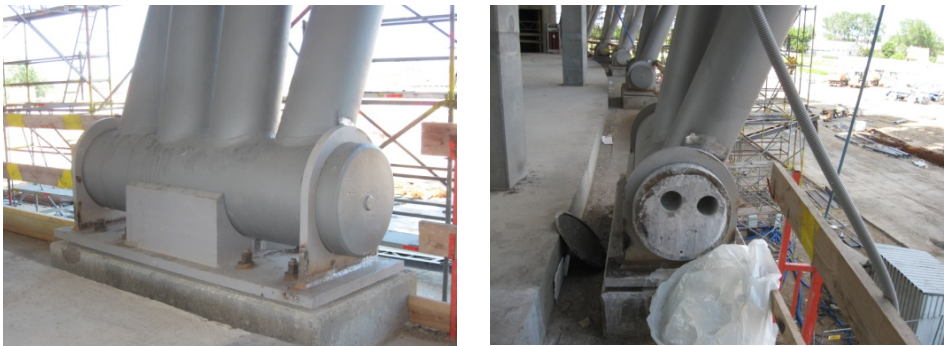
Fig. 14. Support of the girder and the place where the samples were taken
