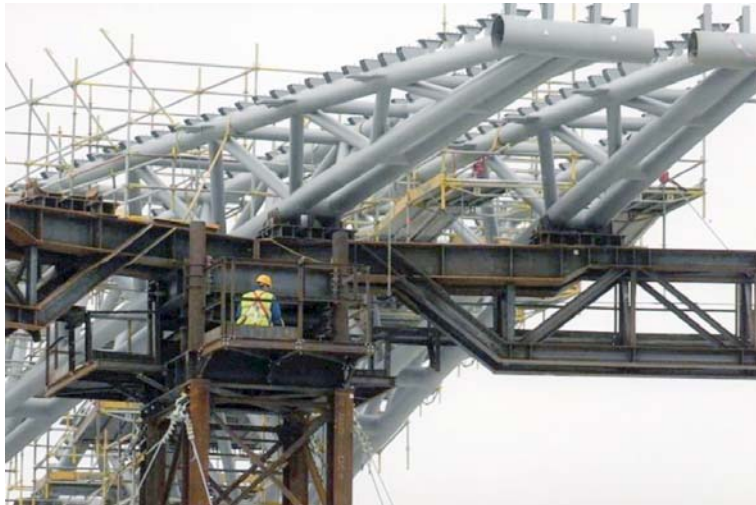
Fig. 19. Tips of two adjacent girders resting on the supporting beam. Components of the main linking ring measuring \phi 500 \times 20 mm can be seen on the girder tips
