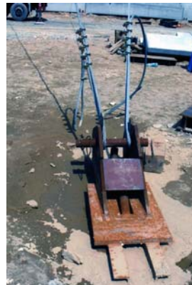
Fig. 12. Anchorage of mounting tower stays within the stadium pitch – a ground anchor (note as for Fig. 11)
