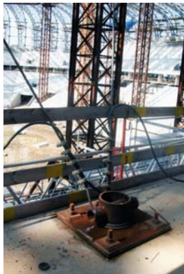
Fig. 11. Anchorage of mounting tower stays to the reinforced concrete structure of the stadium stand (stays of two neighboring towers were fastened to one anchor)
