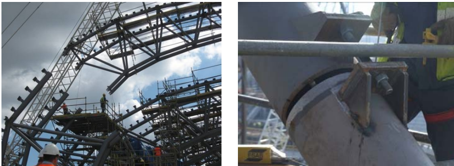
Fig. 13. The connection process of the girder roof part with the facade part
