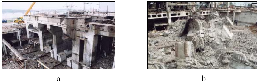
Fig. 1. An example of knocking out of concrete supported structure at Patnow power plant
