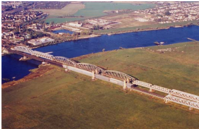
Fig. 7. Present aerial view of the Tczew bridges
