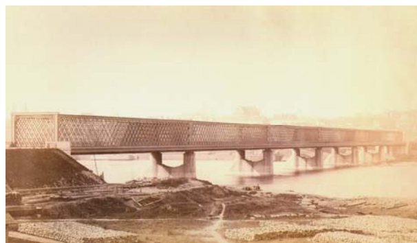
Fig. 3. “Kierbedź Bridge” in Warsaw (1859-1864)
